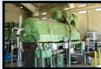
◀ Figure 1. Large Centrifuge used for Separating Solids and Water
